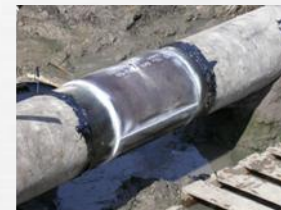
Carry out repairs)
